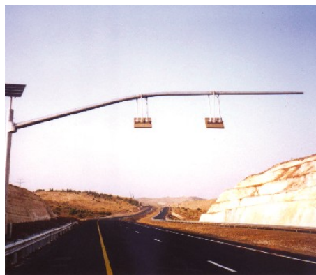
FIG. 2.3 – Cross-Israel highway, with cameras that identify the plate number of the passing cars.
