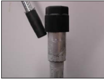
Figure 4.22.a. Detection from the top of a R-134a leak from a MAC system fitting, using a 7 g.yr -1 sensitivity threshold – detector.
