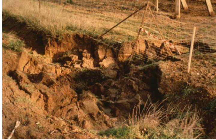
Figure 1. Collapse behaviour in shallow layers of loess directly exposed to climatic actions
