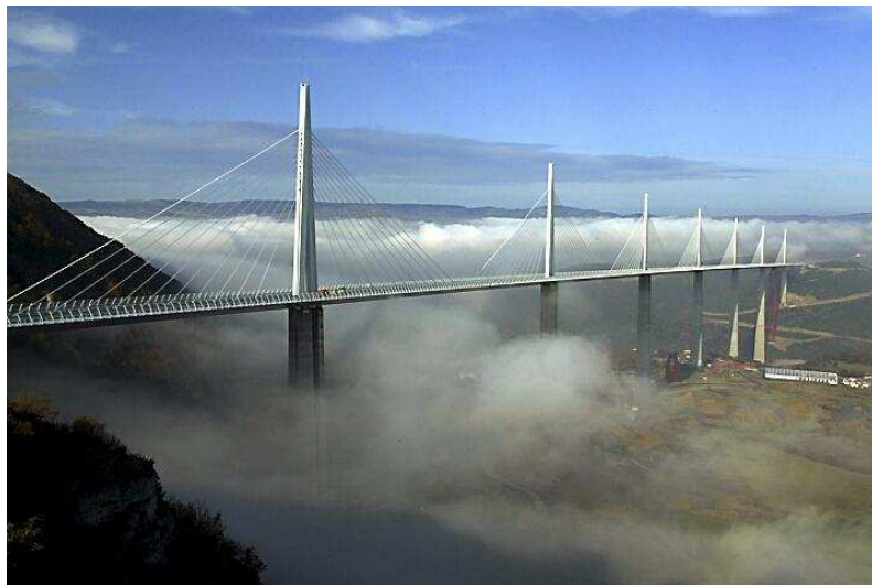
Figure 1: Picture of the "Viaduc de Millau".
