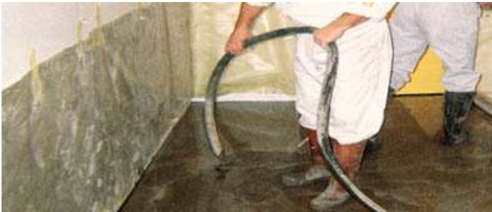
Figure 4.1: Picture of the application of a self smoothing mortar (from [Web11]). To get this property, some adjuvants are added to the basic composition of a mortar, which can modify its drying.
