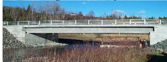
Wotton bridge Wotton 2001, Quebec
