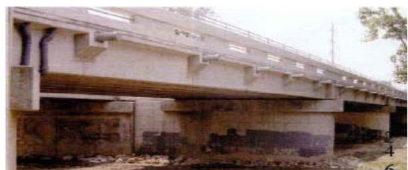
Bridge Street Bridge 2001 Michigan (USA)
