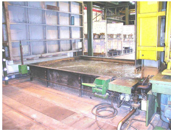
Figure 2.17: (a) Quenching configuration, (b) Industrial water tank agitated by two pumps
