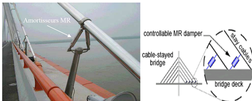
Figure 1.6 – MRF in Dongting bridge in China (after J.M., Ko, Y. Q., and Ni, [13]).
