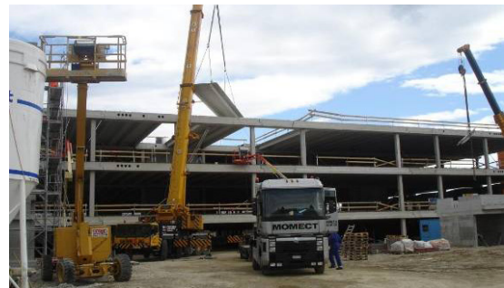
Figure 4-2: Double-tee beams for the construction of an industrial floor
