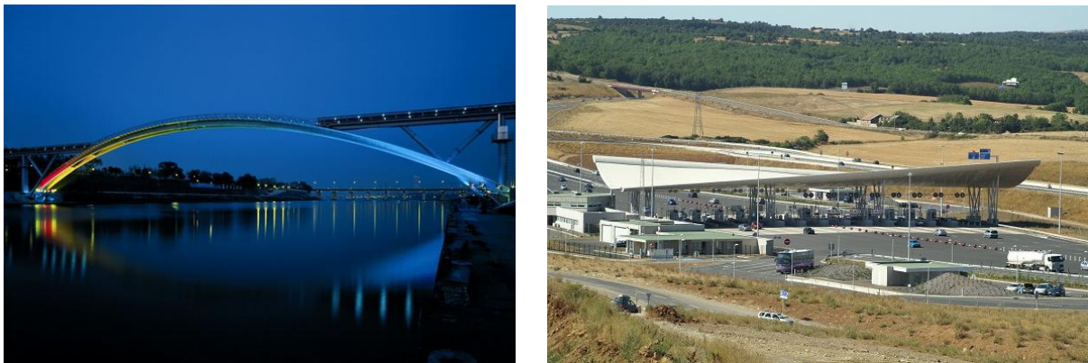
Figure 2-3: Seonyu Footbridge in Korea and roof covering of Millau Viaduct toll-gate in France
