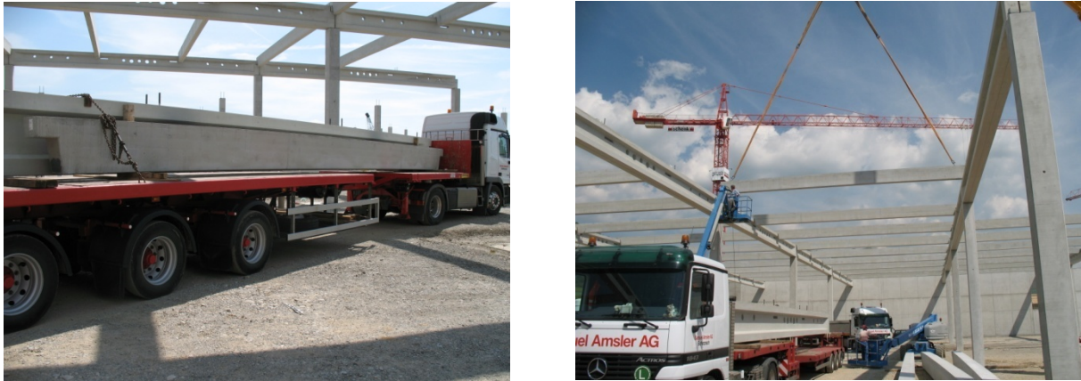
Figure 4-10: Assembly of the precast concrete structure
