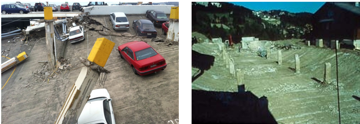
Figure 5-1: Collapses of car parks by punching shear failure in New Zealand after a seism a), in Switzerland due to an overload of embankment b)
