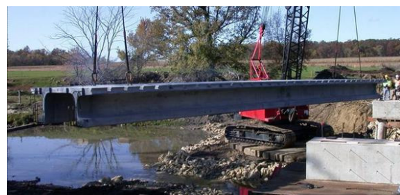
Figure 2-118: UHPFRC bridge girder and construction of Jakway Park Bridge USA
