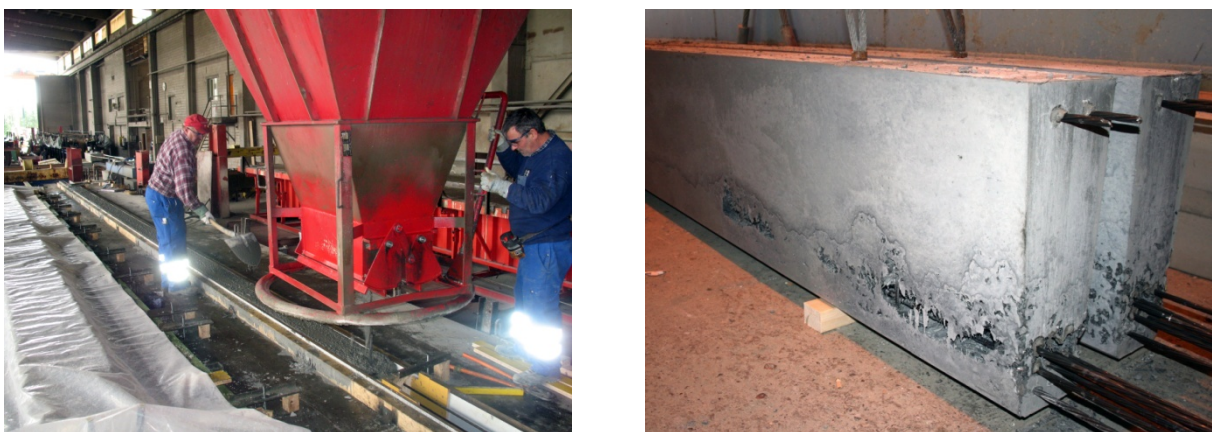
Figure 4-20: Casting process and the first shear beams AV-5 and 6
