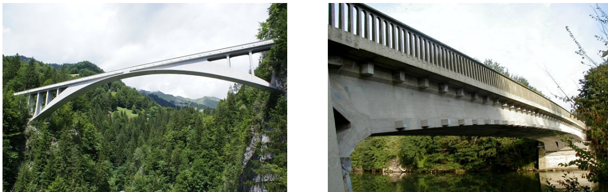
Figure 2-32: Salginatobel Bridge by Maillart 1930 (CH), Luzancy Bridge by Freyssinet 1947 (FR).
