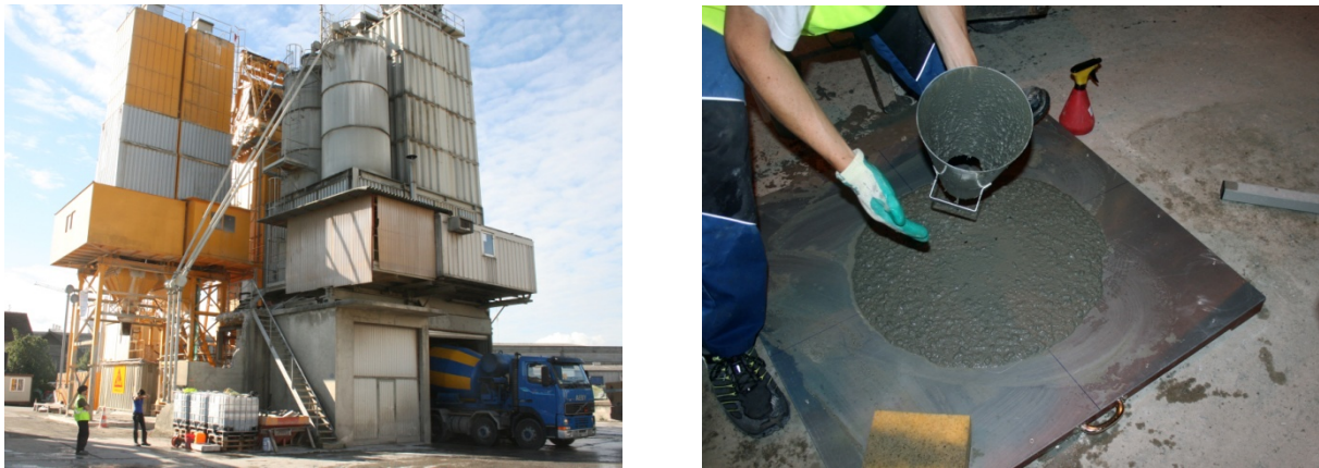
Figure 4-19: Mixing plant and slump flow test before the casting process
