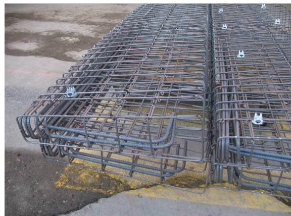
Figure 4-1: Example of precast members and conventional steel reinforcement cage
