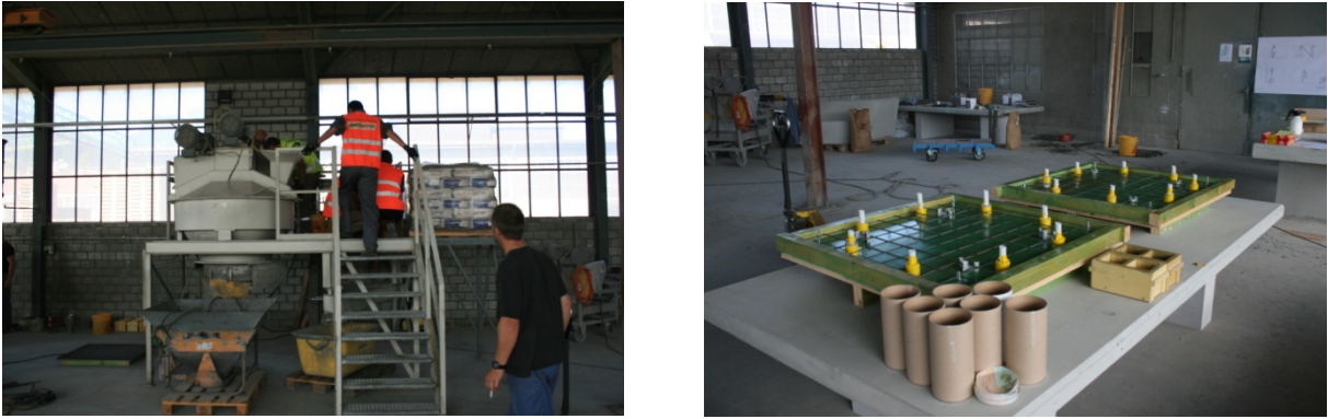
Figure 5-18: Mixer and formworks at Creabeton Matériaux
