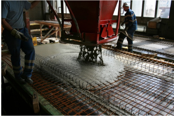
Figure 3-2: Self Compacting Concrete
