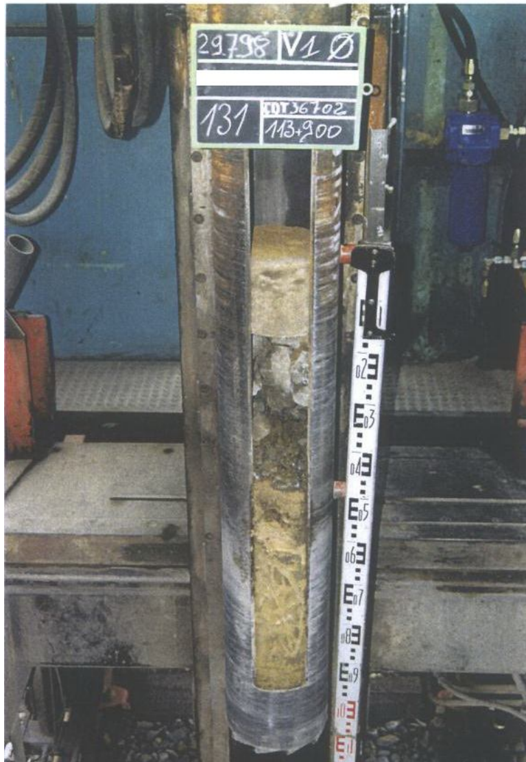
Fig. 10: Core sample from typical ancient railway sub-structure
