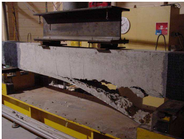
FIGURE 1.3 – Rupture par peeling-off (Dallot, 2007)
