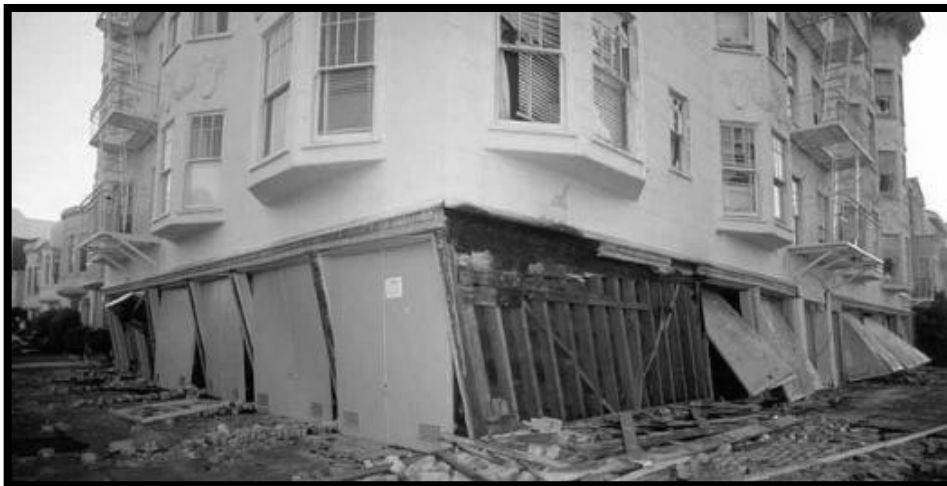
Figure 41 -A soft-story building damaged after the 1989 Loma Prieta earthquake. Source: California Watch.
