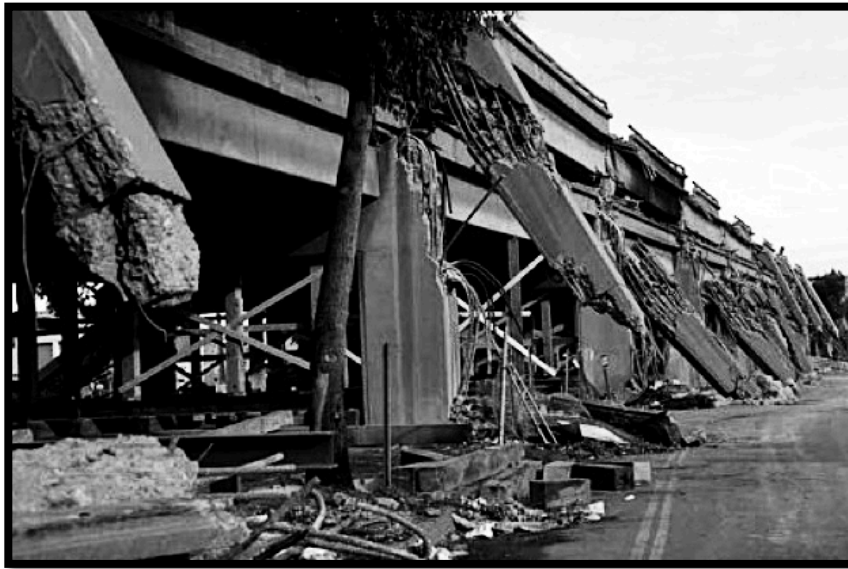
Figure 16 - The Cypress Highway after the 1989 earthquake. (Source Wikipedia)
