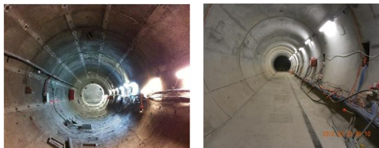
Fig. 2. 2. GCR section. Flexible support (left) and final lining installed after 7 months (right)
