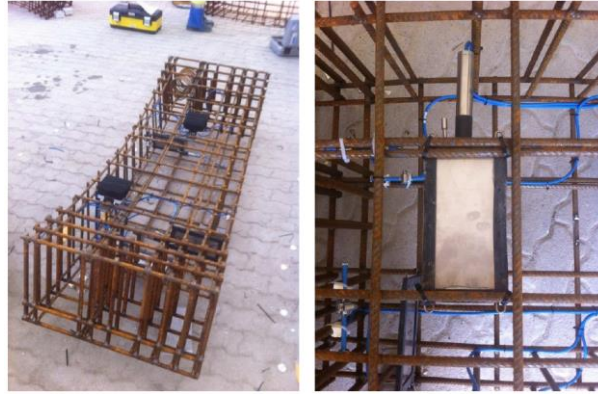
Fig. 1. 16. Implementation of measurements gadgets in the segments before the concrete is poured
