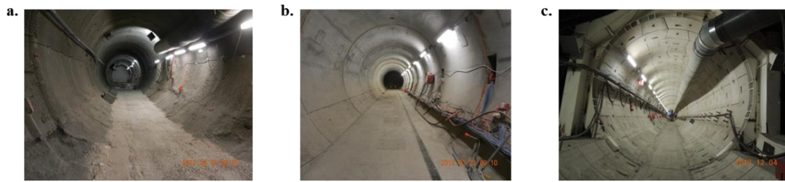
Fig. 1. 7. Rigid support installation: a. Support of 45 cm of fiber shotcrete (BEP drift). b. Support with 20 cm of fiber shotcrete and a permanent lining installation 7 months after (GCR drift). c. Support composed of rings of prefabricated segments (GRD4 drift)
