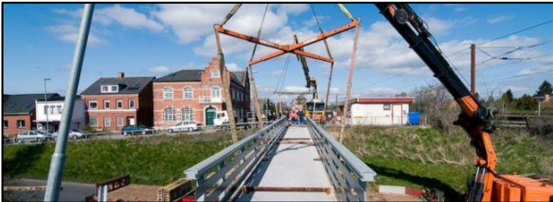
*Figure 1.1: Construction of a pedestrian bridge NørreAaby, Denmark 2007 extracted from FRP structures scientific and technical report 2014*
