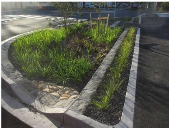
Figure 6 : Stormwater biofilter (Payne, 2017)
