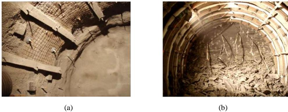
**Figure 1.5** : support systems for GCS (a) and GED (b) drifts. (from [42] and [93]). Supports are mainly composed of radial bolts (HA25 of 3 m length), with a ~15 cm of fibres shotcrete and welded mesh.
